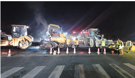
S515枣薛线与S322枣欢线路口坑槽修补
